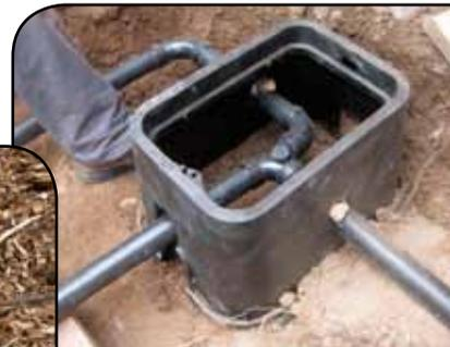
Above. A laundry greywater system uses pressure produced from the machine to push water out to fruit trees.
