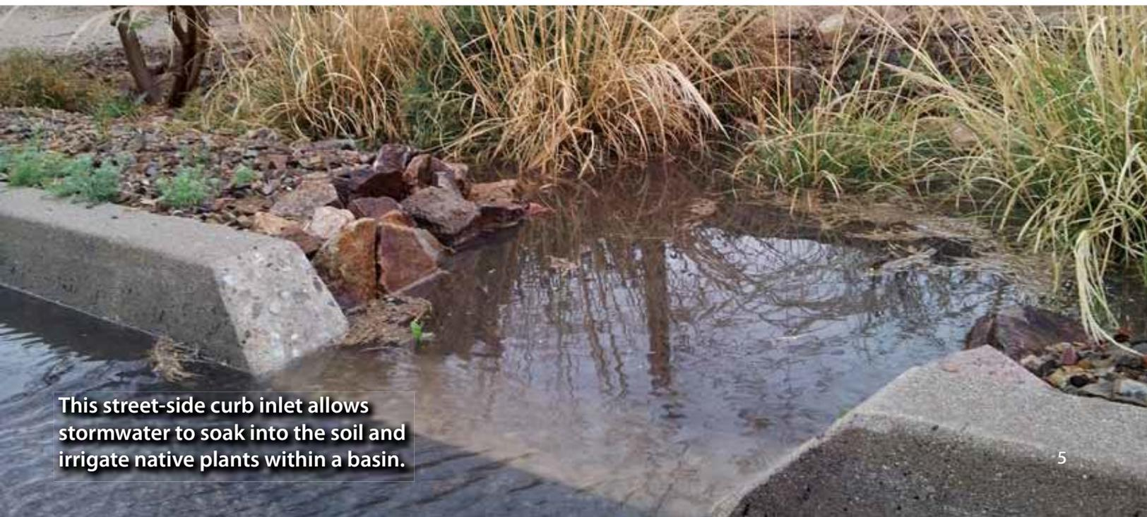
This street-side curb inlet allows stormwater to soak into the soil and irrigate native plants within a basin.
