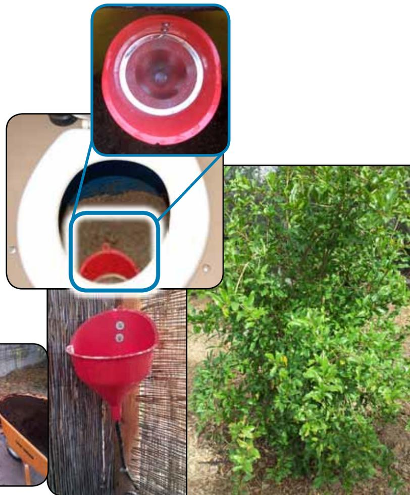
From top. A urine diversion funnel directs urine below ground to infiltrate directly into the soil. Urine diversion can be placed within the barrel and as a separate male urinal. To reduce salt build-up, flush the soil with rainwater or greywater when possible.
