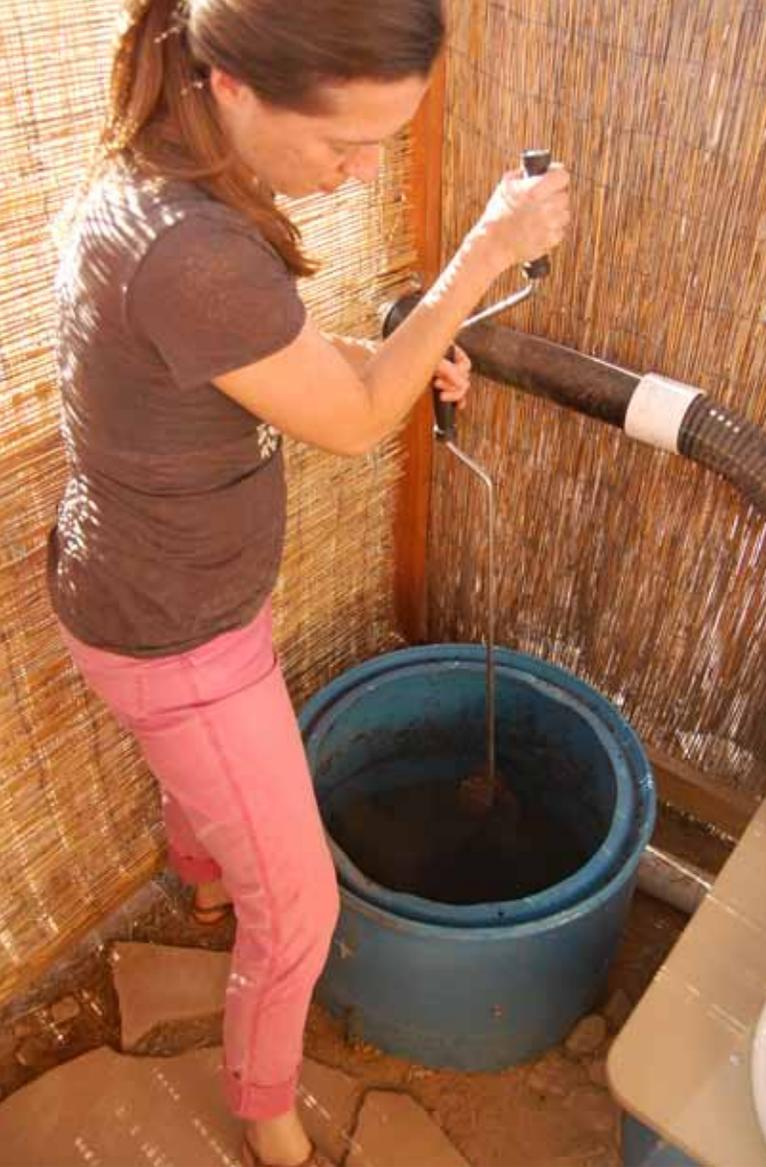
*The composting toilet is easily aerated with a compost crank.*
