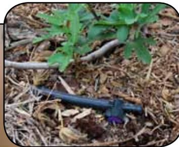
Below. Gravity-based branched drain distributes shower/sink water to basins.
