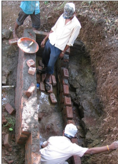
Spring box installation.
