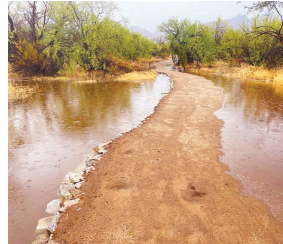
Restoration efforts included creating raised earthen trails to shed water into nearby basins. In addition, rogue trails were closed to reduce wildlife habitat fragmentation.
