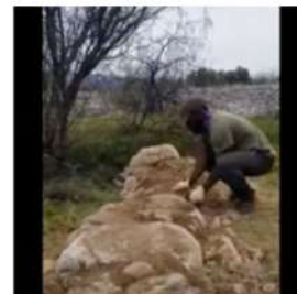
Steward In Place: A Day In The Life: Restoration Team
