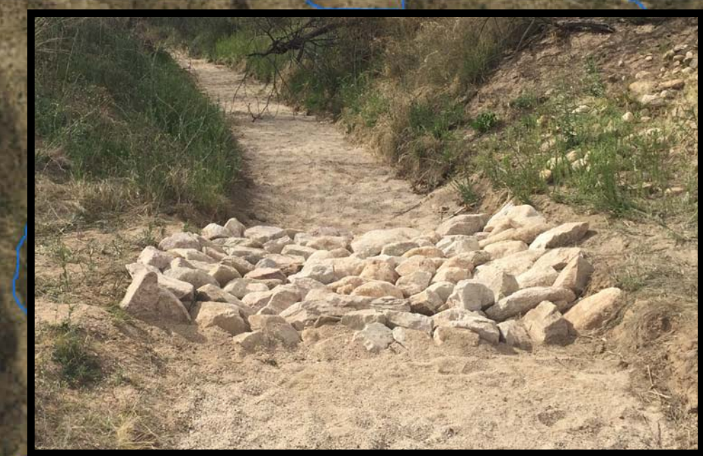
A one-rock-dam restores degraded arroyos and slows stormwater flows which may enhance aquifer recharge.
