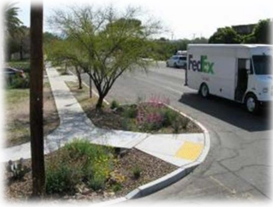
Figure 6. Street: Asphalt removal for creation of in-street basins to narrow roads, slow traffic, and harvest street runoff.
