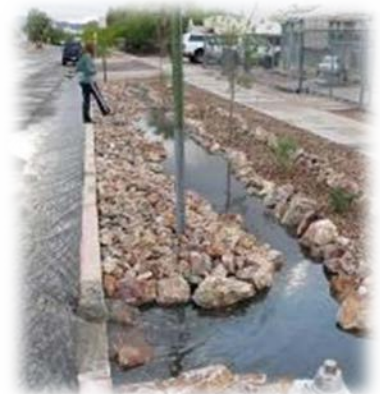
Figure 4. ROW: Rain gardens behind the curb with curb cut inlets to harvest water from the street
