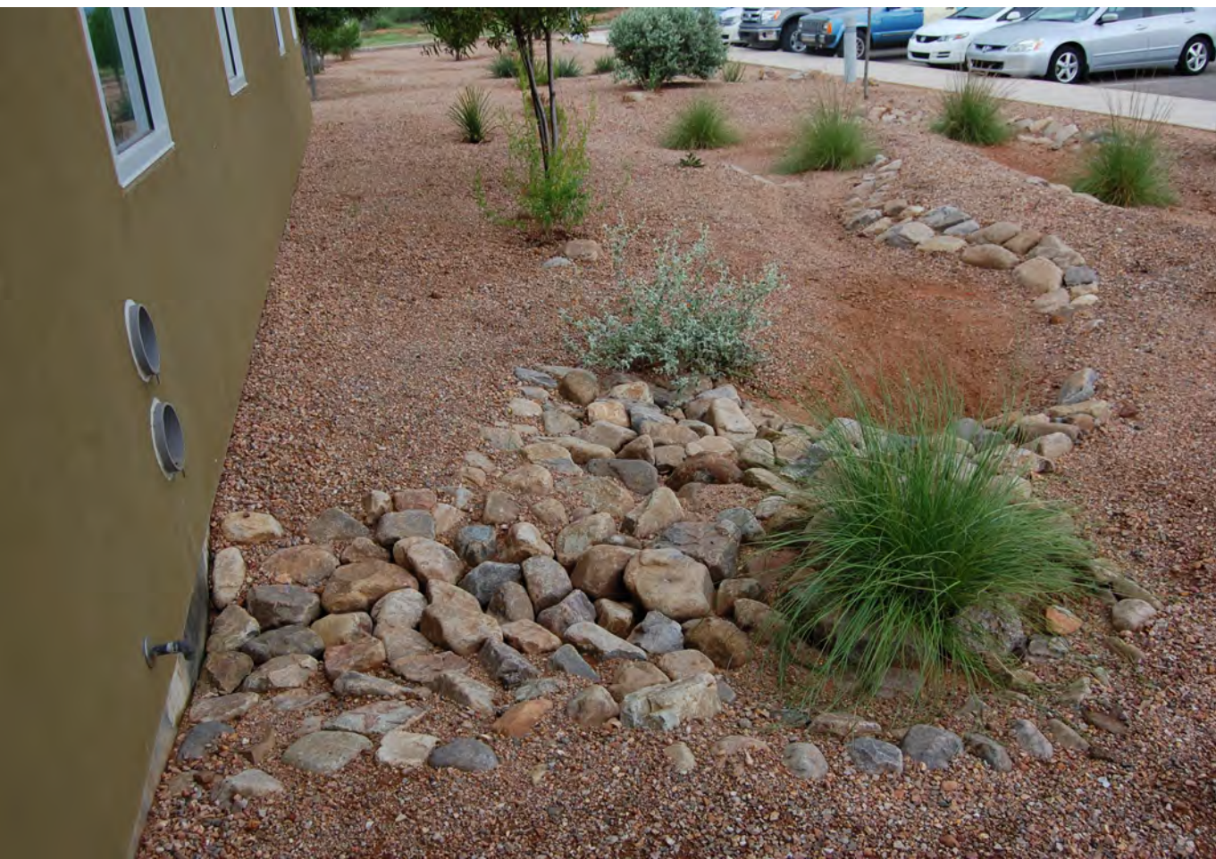
Left: A raingarden retrofit near the Student Union of Cochise College's Sierra Vista Campus guides rainwater from the downspout through the landscape in a series of swales and basins. This feature helps to reduce nuisance flooding by infiltrating it into the soil to benefit the plants.
