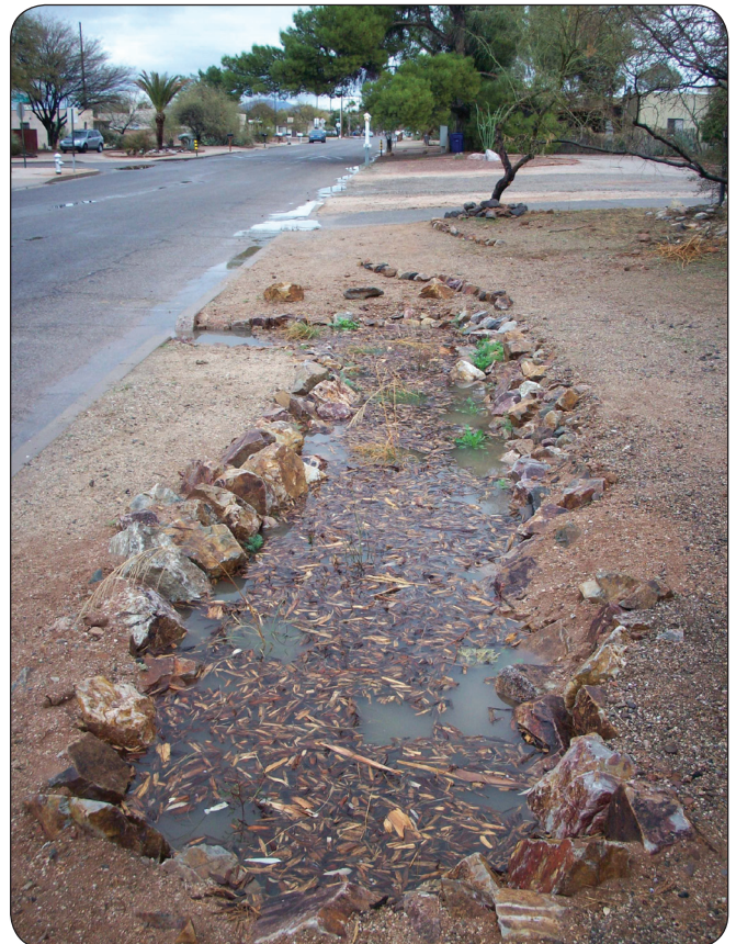
Narrow basins with steeper sides will need rockwork to stabilize slopes. This basin is capturing storm water off the street.
