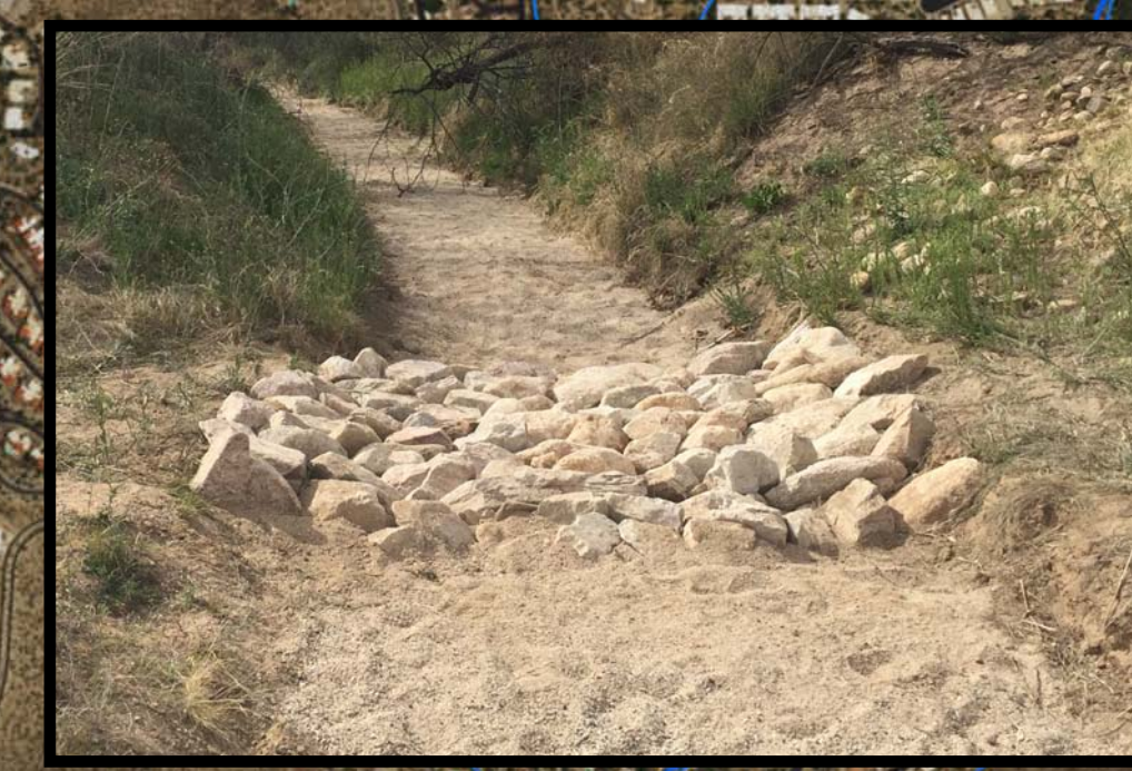
A one-rock-dam restores degraded arroyos and slows stormwater flows which may enhance aquifer recharge.
