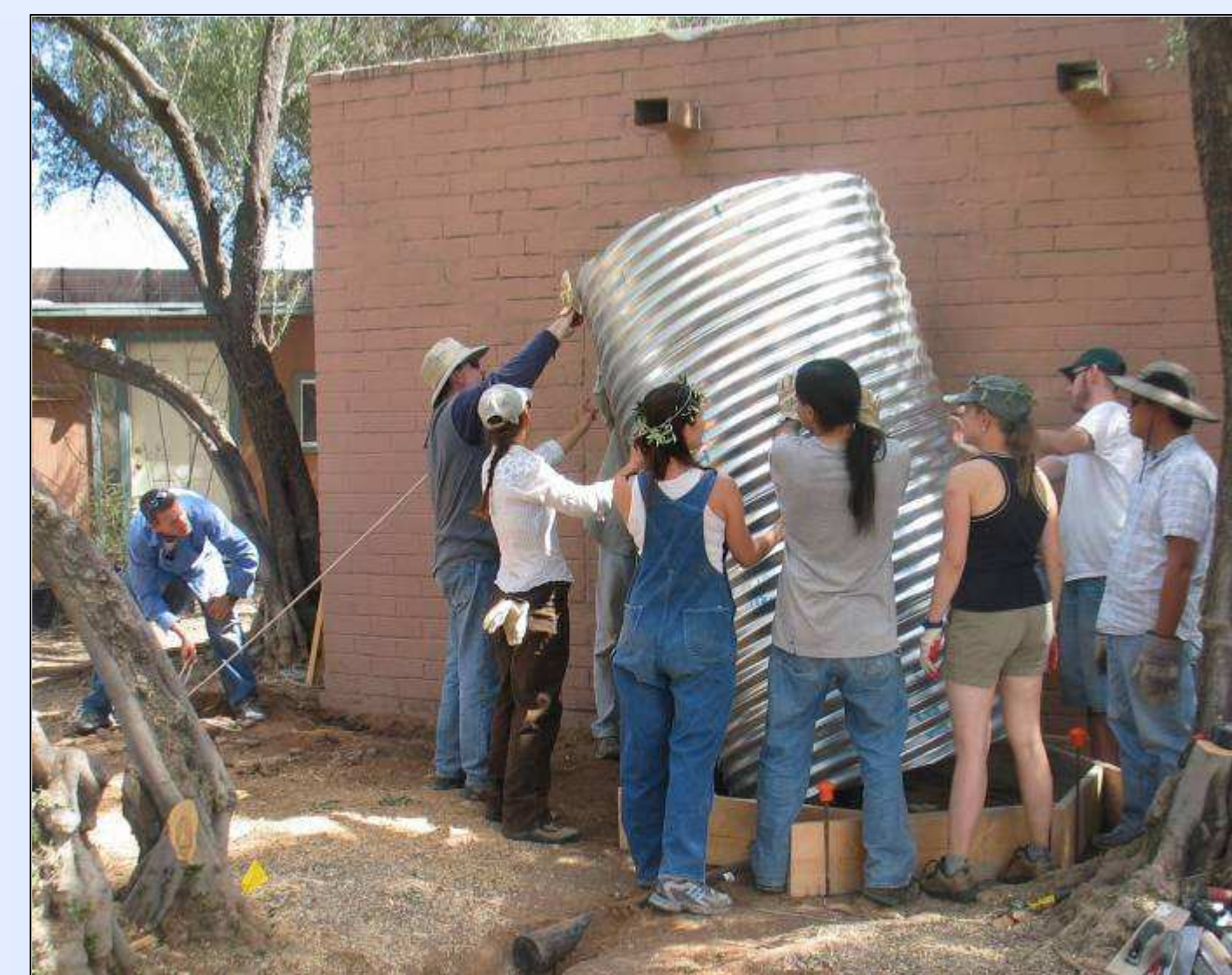
Site: TNC, workday – cistern installation
