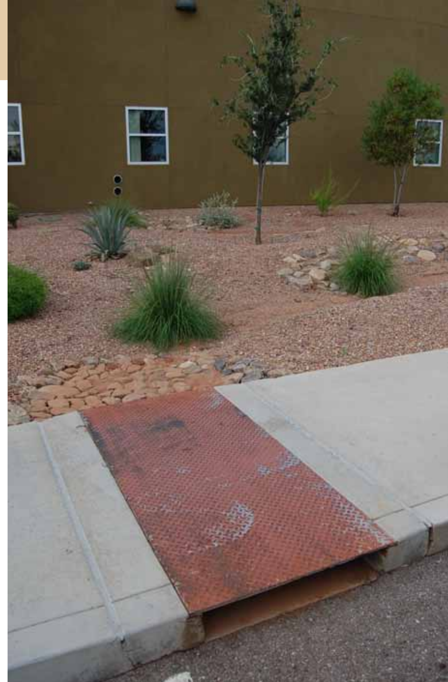
Variations of sidewalk scuppers allowing stormwater to flow under sidewalk.
