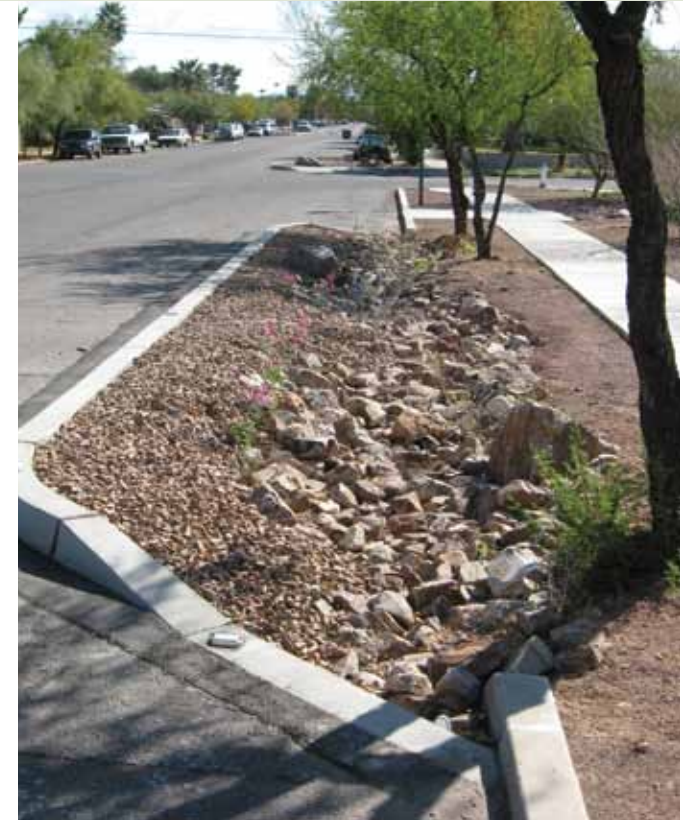
In this just-installed chicane, 4"-8" rip-rap is used in the channel where stormwater will flow rapidly, and 1" gravel covers upslope areas.
