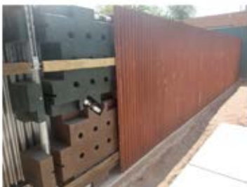
1,000 gallon patio wall built with Rain Blocs.
