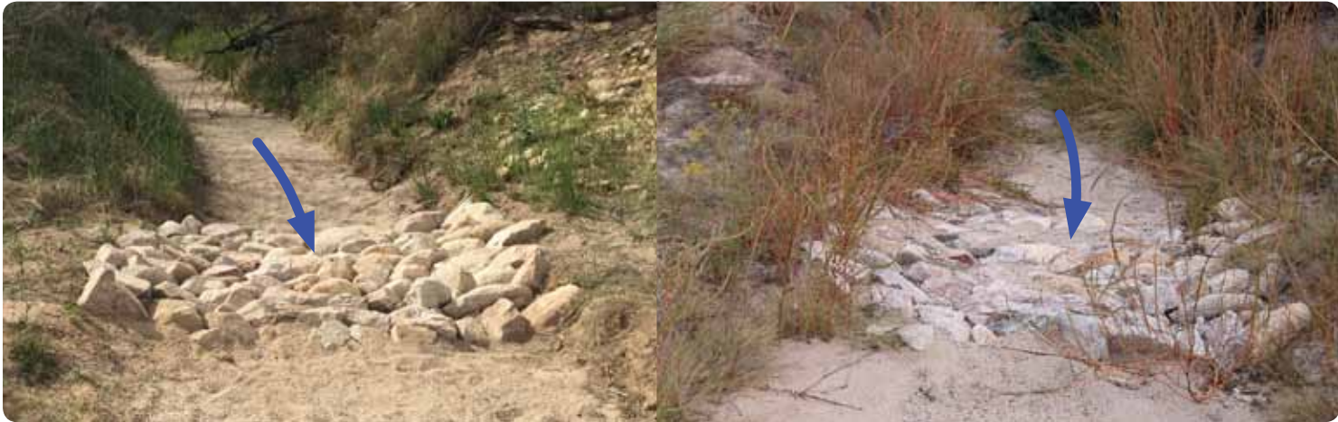
Left: A one rock dam as part of a series to treat an incised arroyo flowing into Lower Sabino Creek, March 2016. Right: The same one rock dam following summer rains with an increase in sediment, Oct 2016.
