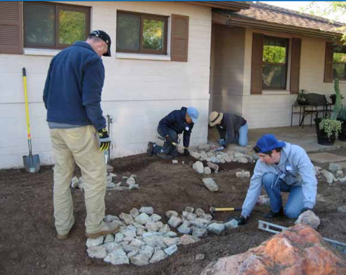
Green Living Co-op members placing rocks in a swale to convey rainwater from a downspout to a rain garden basin.
