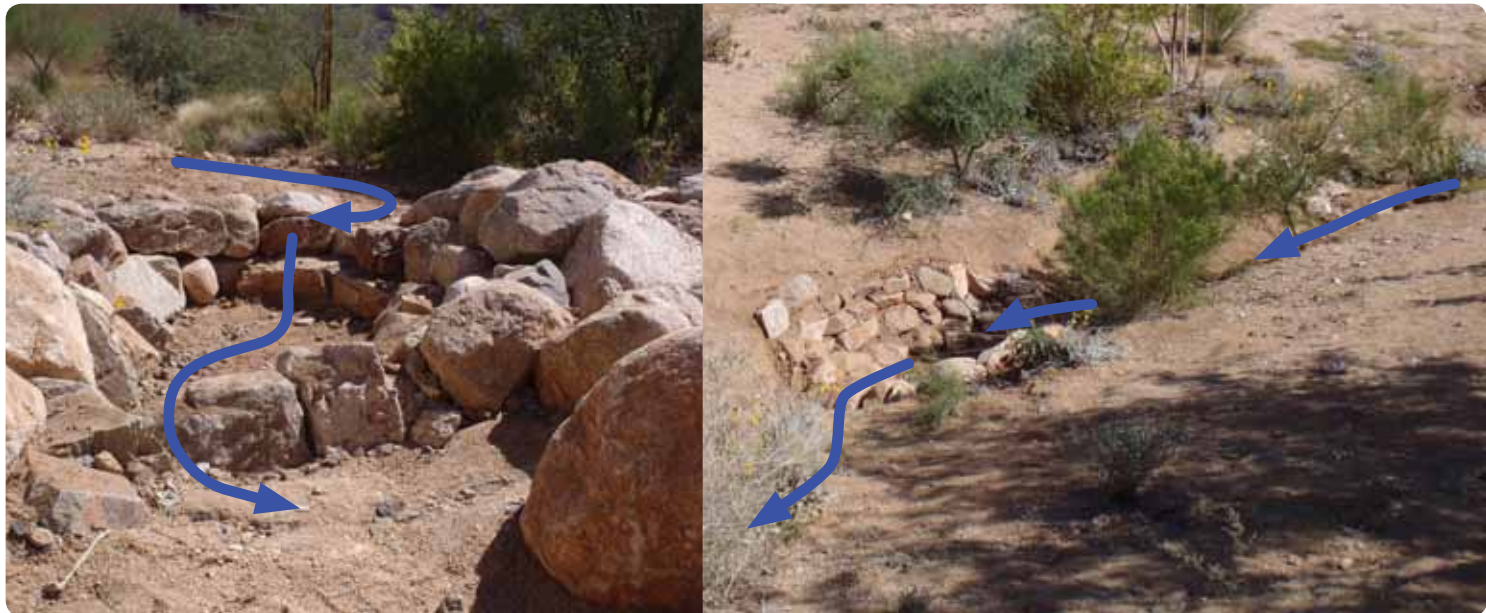
Left: A Zuni Bowl looking upstream. Right: Another Zuni Bowl showing placement within the same gully.
