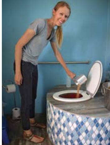
Masonry chamber composting toilet
