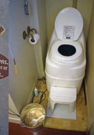
Sun-Mar composting toilet
