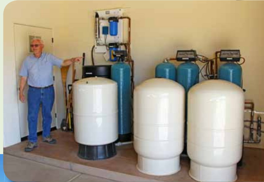
A filtration system cleans stored water for potable use
