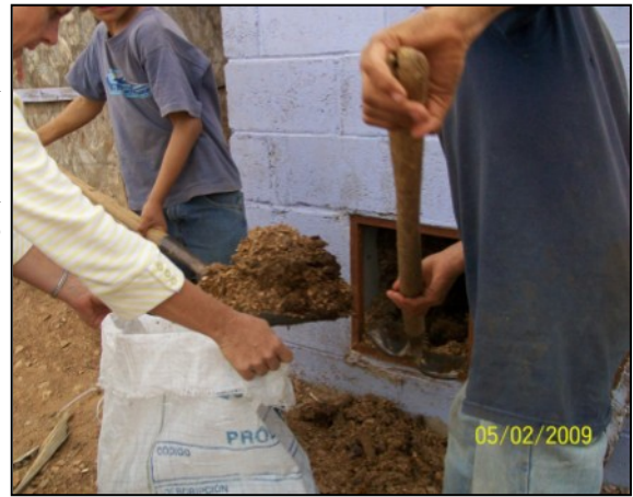
Removing finished compost from toilet
