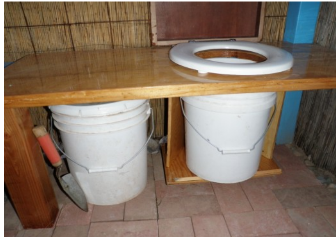
Simple outdoor composting toilet (right) with mulch clippings bucket on left. When 5 gallon bucket is full, it is added to a larger humanure compost pile.
