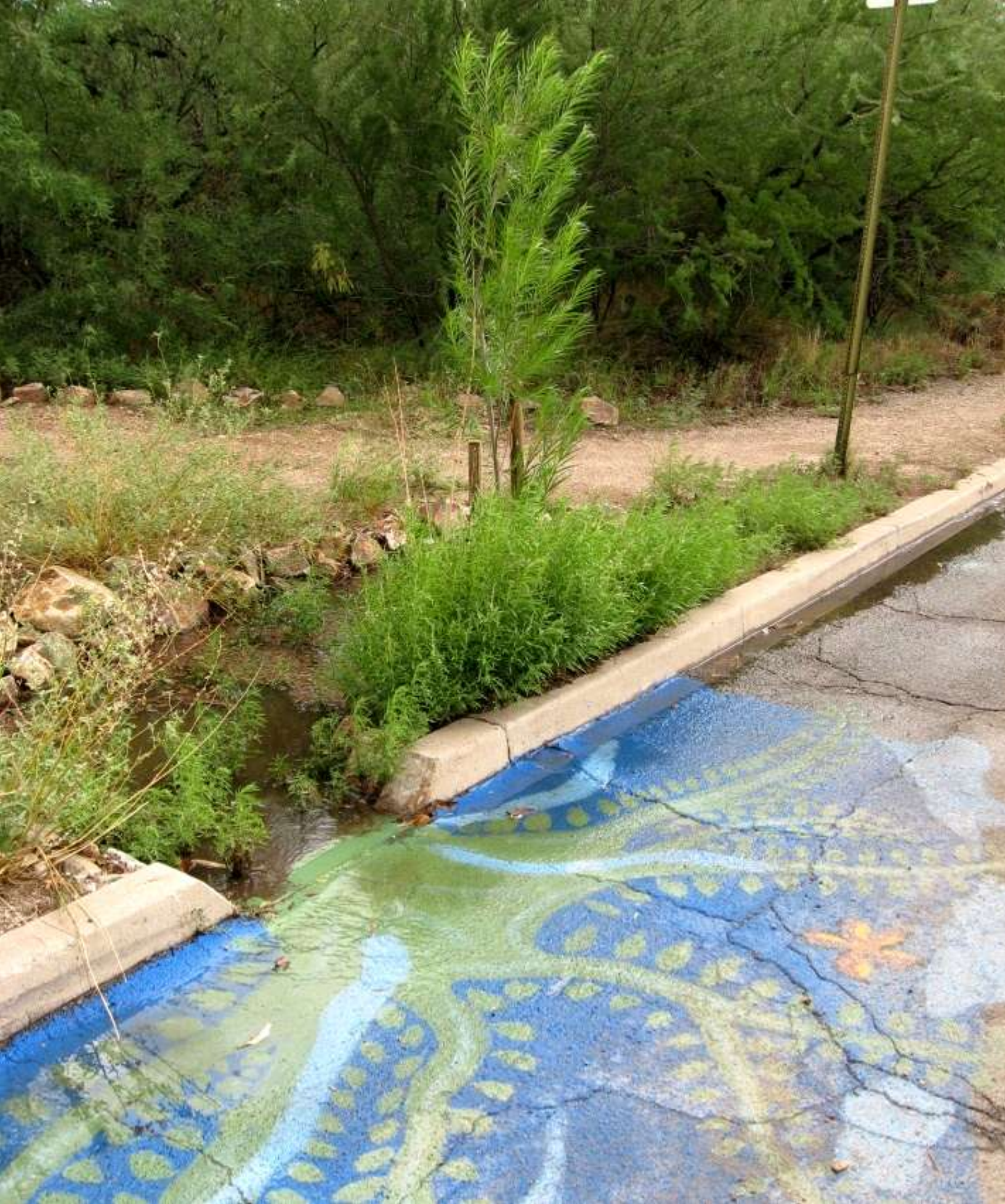
Stormwater runoff from neighborhood streets flows through curb cuts into vegetated basins, passively irrigating young trees and cleaning the stormwater of pollutants through natural processes.
