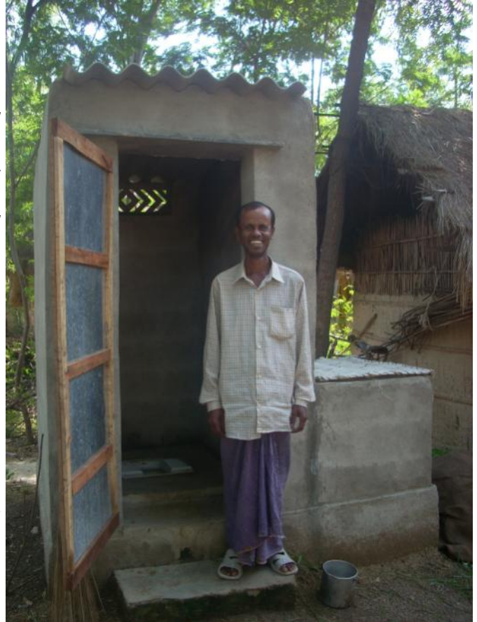
Adhivas Mandal, a villager from RH3, stands outside his newly constructed double pit composting toilet.
