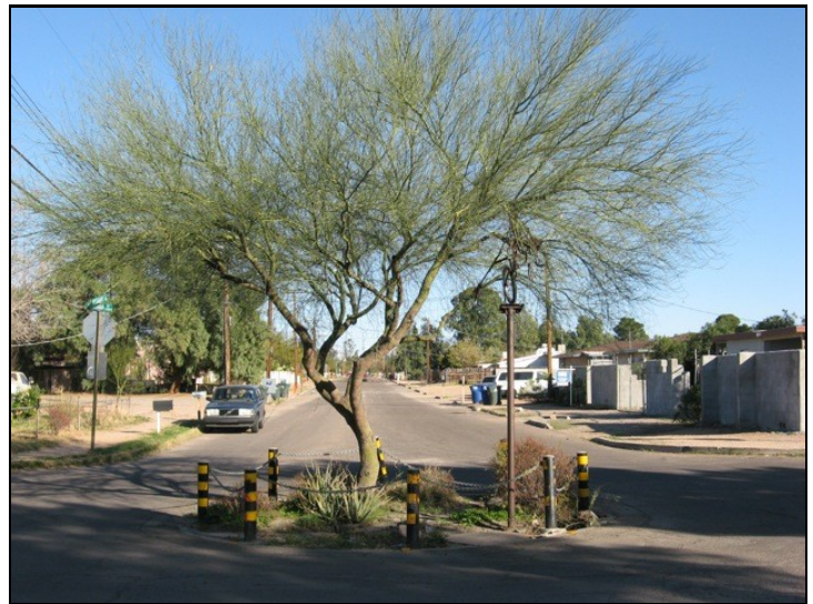
This water harvesting traffic circle reduces heat-trapping hardscape; and its vegetation provides shade, stormwater treatment, beauty and wildlife habitat.
