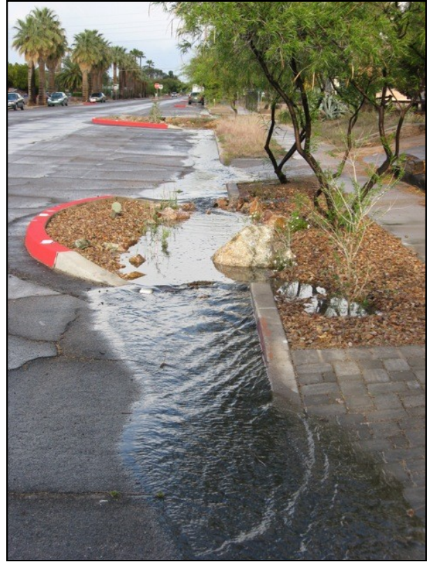
This just-planted chicane in Rincon Heights neighborhood slows traffic by reducing street width, and helps treat stormwater by slowing and infiltrating some of it in vegetated areas.
