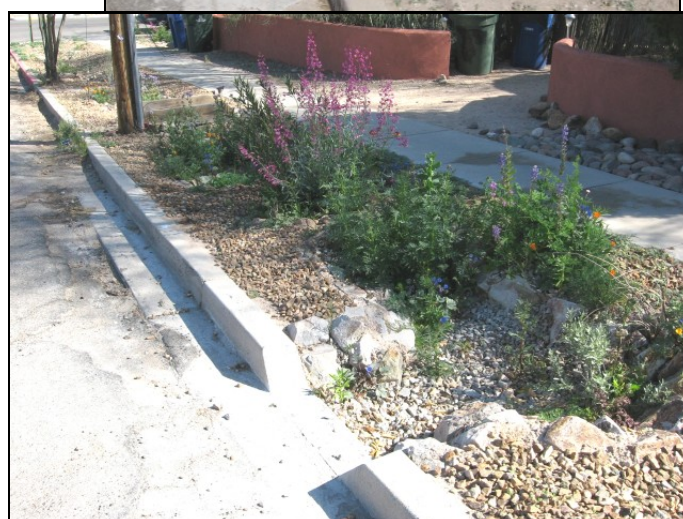
A right-of-way in Rincon Heights neighborhood before (above) and 5 months after (below) installation of curb cut, basins and plants.
