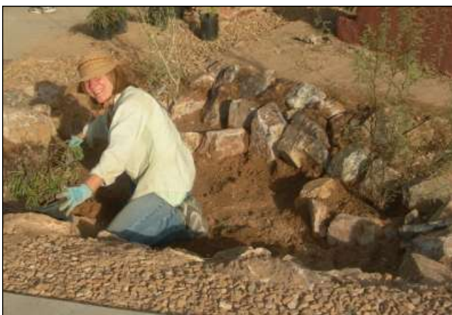
Volunteer plants native shrub in newly created rainwater basin.
