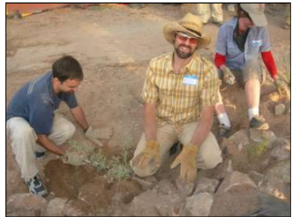
WMG volunteers plant Tucson basin native plants in newly created basins in the public right-of-way.
