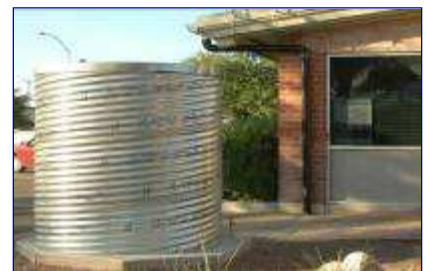
Rainwater harvesting cistern used to store water runoff from roof.
