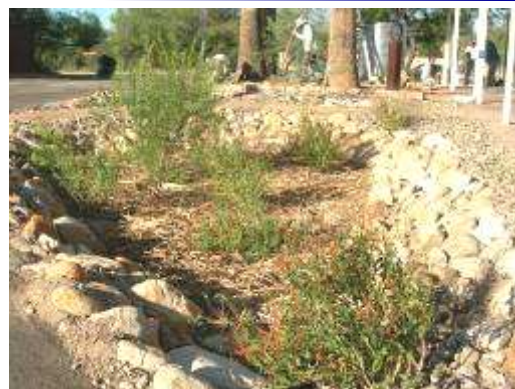
Rain water harvesting basin in front of Ward III City Council Office, Tucson, AZ.
