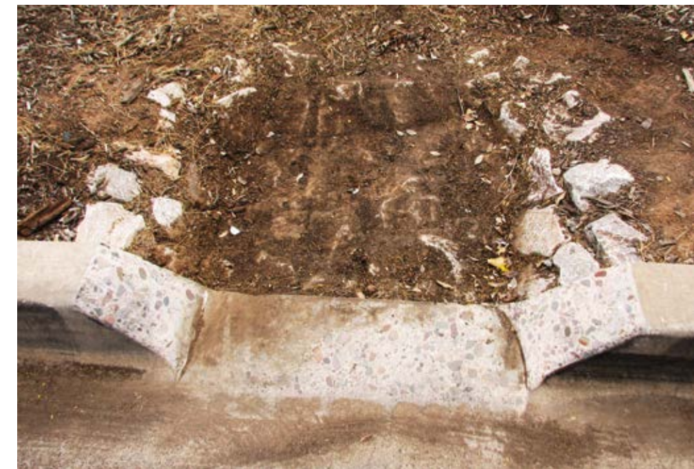
Top Right | Recently installed sediment trap—a rock apron set adjacent to the curb cut to capture sediments in stormwater before moving into the basin. Bottom Right | Sediment needs to be removed occasionally from sediment traps, as was done in this basin.
