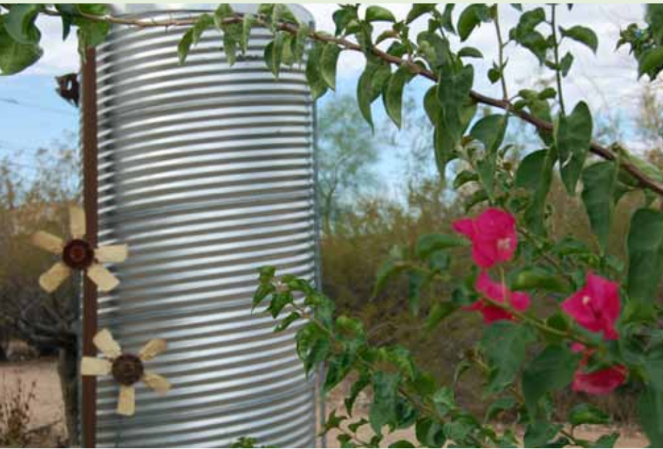
Steel cistern captures roof runoff to water landscape
