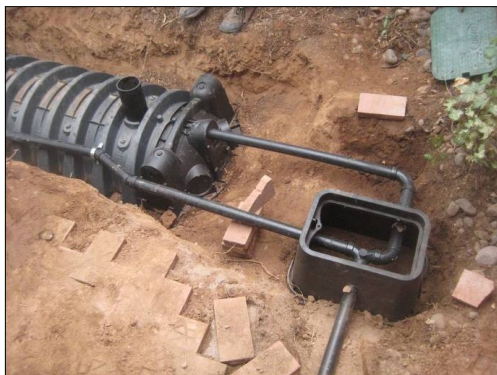
Greywater flow is split using a double ell in the valve box and distributed to each end of the infiltration chamber.
