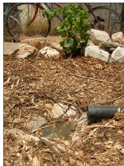
Greywater discharging into a mulched basin.
