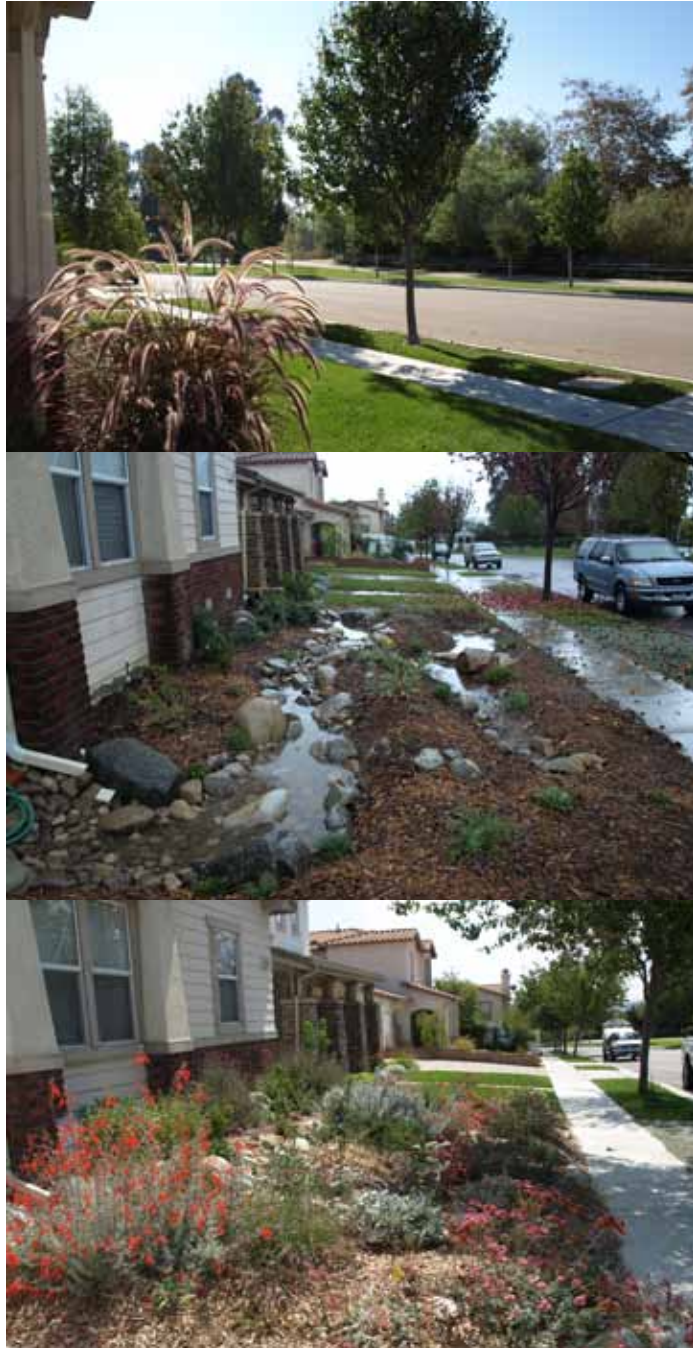
Stormwater-capture Transformation: A downspout at the corner of this Ventura, Calif. residence once flooded water downslope to the street. After a Ocean Friendly Gardens workshop, earthworks captured water in the yard—supporting a lush garden the following year.
