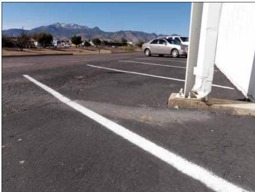
Downspout to Nowhere: This downspout is typical of lost opportunities to reap the benefits of stormwater, as it pours out into a parking lot and drains into a neighboring wash—without feeding into shade-providing, habitat-supporting desert landscapes along the way.
