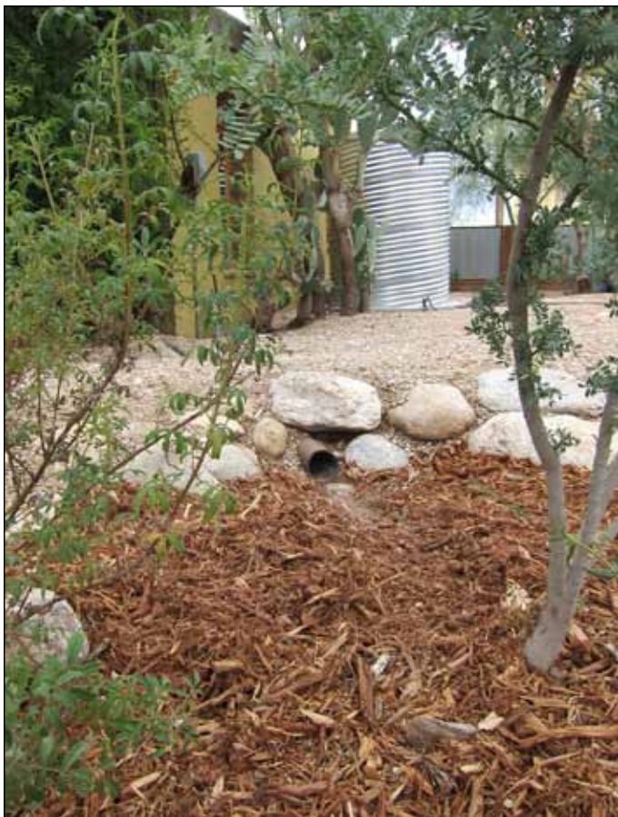
A downspout that once emptied next to a residence's foundation now directs water to a young ironwood tree and other native plants, while a downspout-fed cistern provides water to other young native trees, plants and wildflowers.
