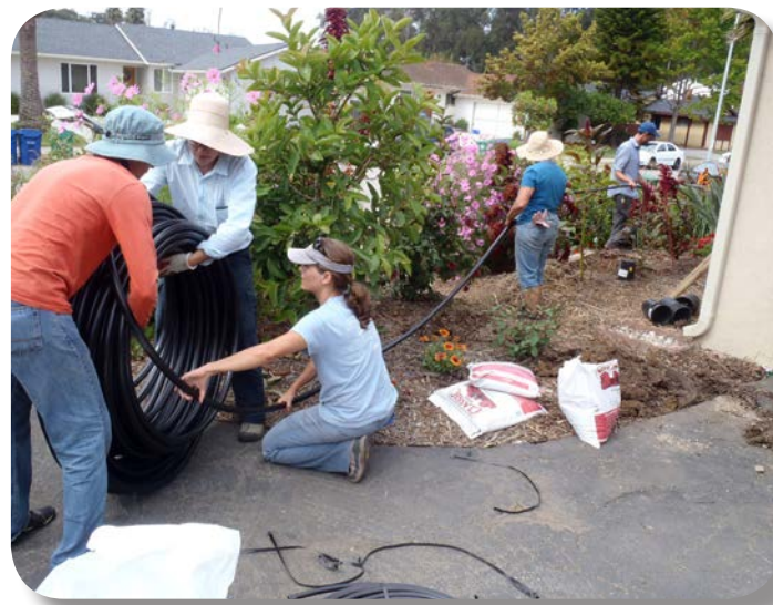
Volunteers install a subsidized greywater system through a WMG workshop in Santa Barbara, CA.
