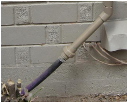
Closeup of cleanout connection option with 1" PVC union to barbed adapter for transition to 1" poly line
