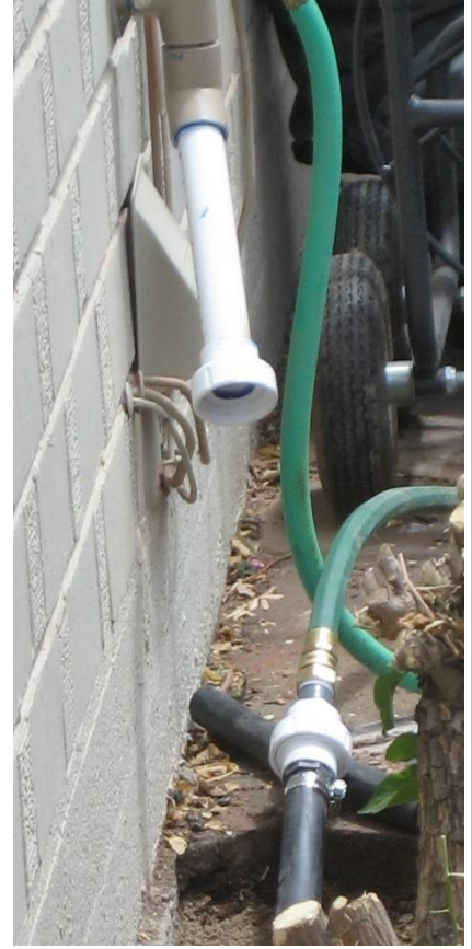
Cleanout option disconnected from laundry diversion to flush line with hose.
