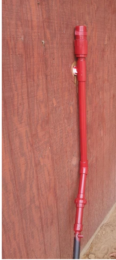
PVC painted to protect from UV degradation with hose cleanout option.
