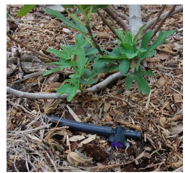
1/2" adjustment valve outlets into mulched basin near fruit tree.
