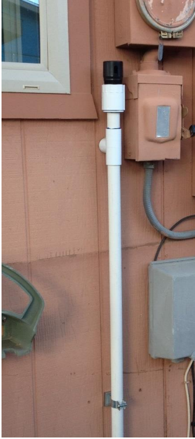
1" PVC stubout from inside laundry diversion with anti-siphon/vent
