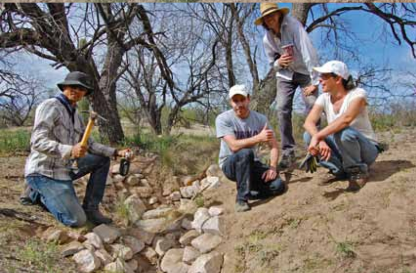
Trainees worked with Trevor Hare to build a media luna (top) and a Zuni bowl (bottom right), rock structures to reduce erosion and infiltrate rainwater in this Sabino drainage. Bottom right: Catlow Shipek meets with Michael Woodin to assess restoration opportunities.
